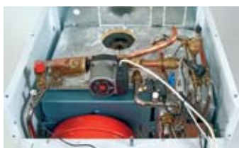
Pipework connections [aerial view] highlighting drop-down control panel.
