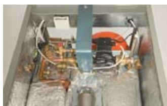
Flow, return, hot and cold valve connections
